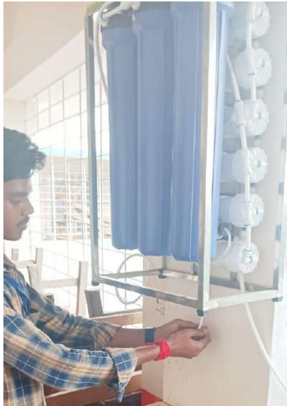
Water Filter Installed at 2 nd Floor
